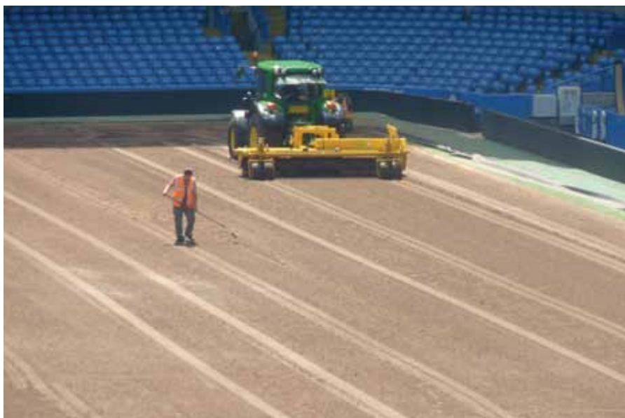
80 tonnes of sand was applied to the 7,000m 2 pitch area
